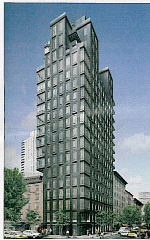
The Isis Condominium is an 18-story condo tower currently under construction on Manhattan's Upper East Side in New York City.
